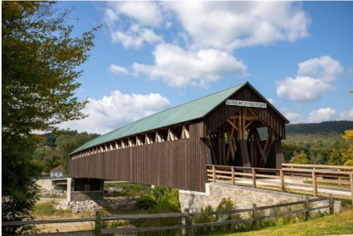
This covered bridge was one of many scenic checkpoints selected by our Rally Master, Ken Relation Story on page 5
